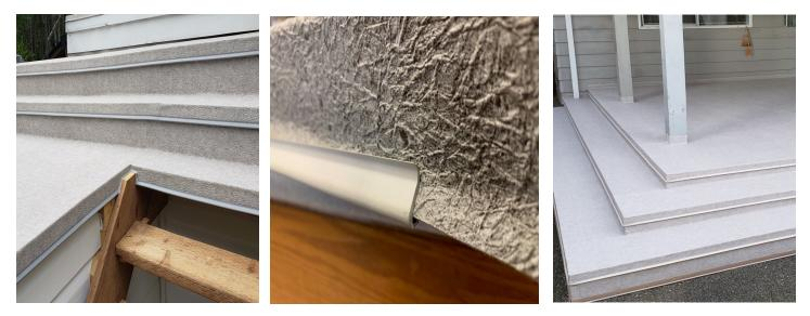
One of the most common issues with the standard U-Channel clip design is that in extreme cold/hot weather conditions, the standard clip would **FALL OFF** or sag on the flashing causing a service callback .
